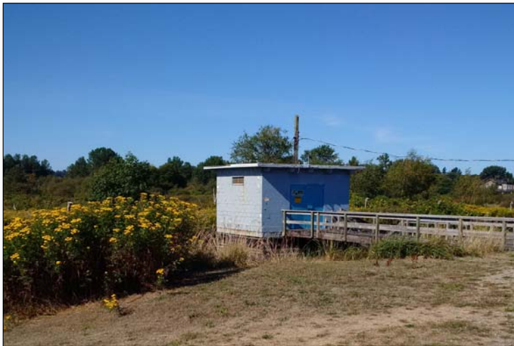
Existing Pump Station
