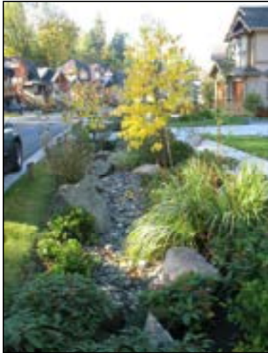
Bio-Retention Swale
