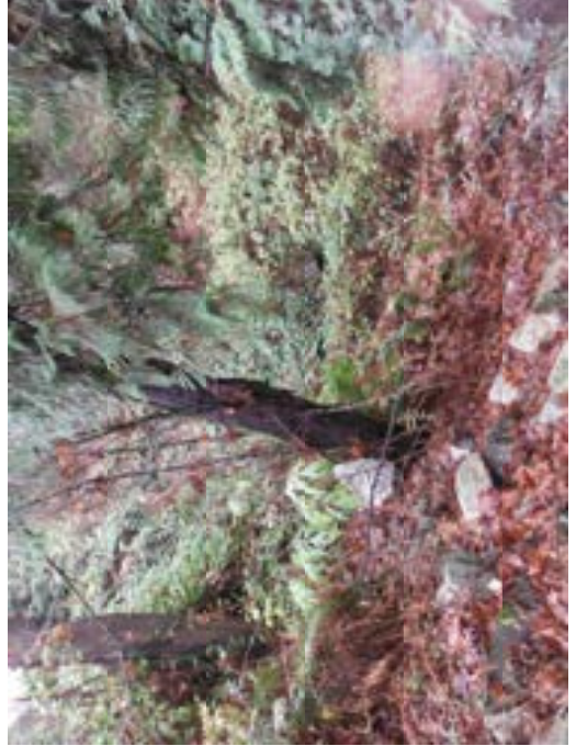
PHOTO 16 – Rip rap slope below Main Street
