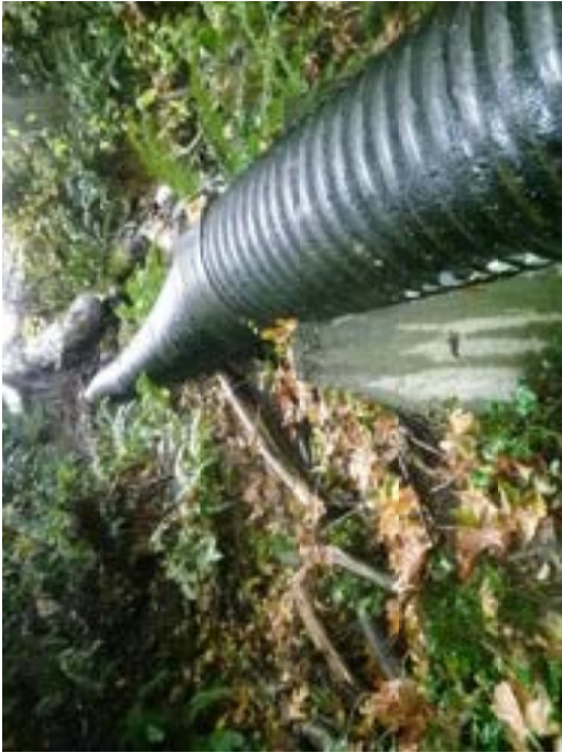
PHOTO 13 – Pipe leading to outfall east end creek
