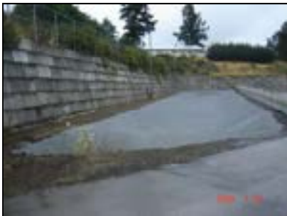
Surface Infiltration Swale
