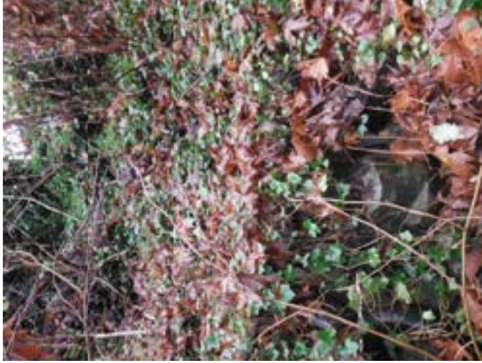
PHOTO 6 – Tire and rock constructed slope, downslope River Road
