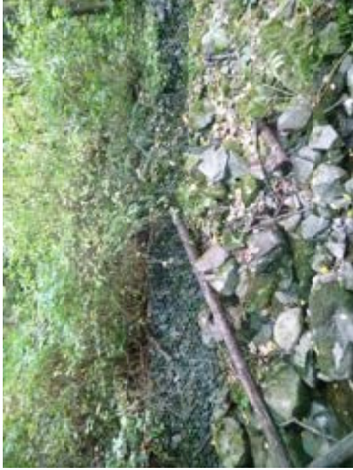
PHOTO 30 – Gabion walls below outfall
