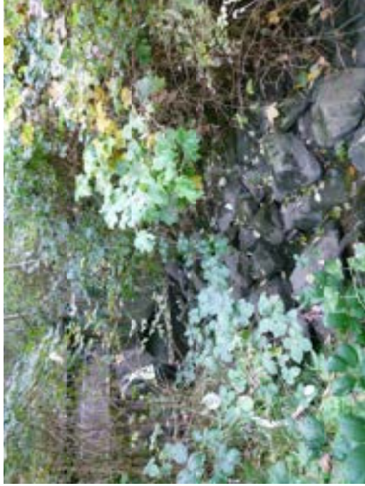
PHOTO 14 – Rip rap above culvert inlet at Nordel Way
