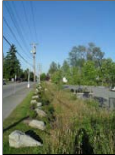
Bio-Retention Swale
