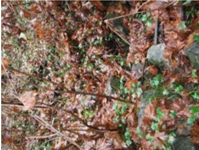
PHOTO 5 – Rip rap below River Road
