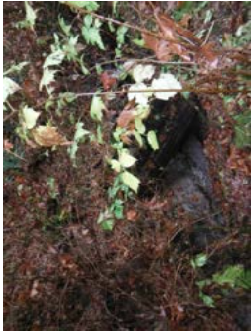
PHOTO 7 – Stump in creek, potential blockage
