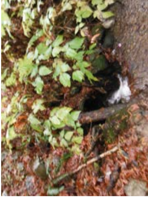
PHOTO 2 – Another outfall, east end ravine
