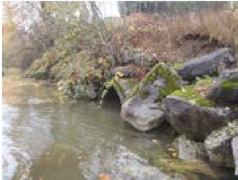
Culvert at the mouth of Nelson Creek
