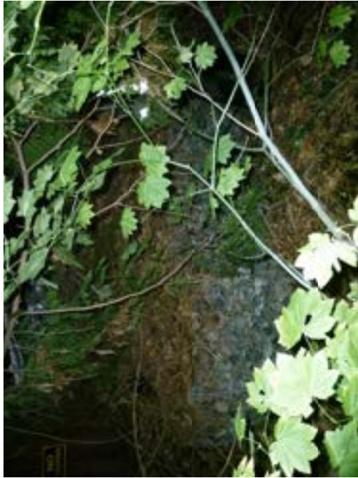
PHOTO 5 – Gabion wall, north bank
