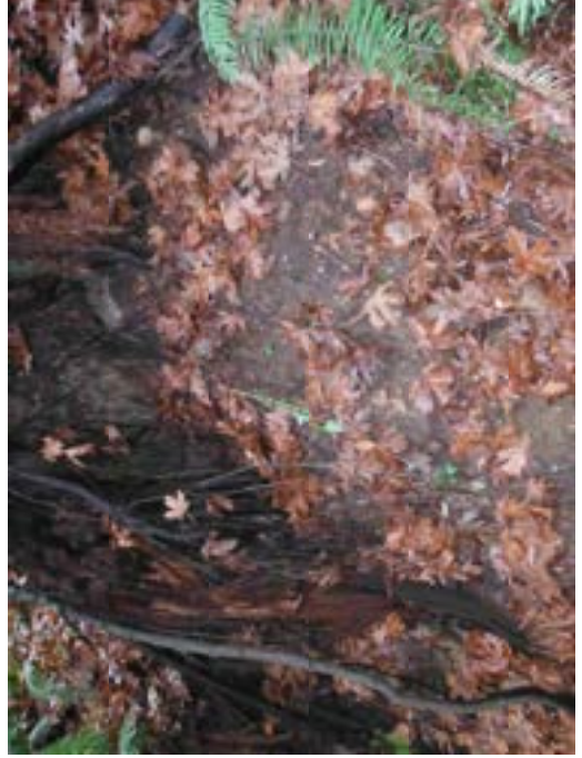
PHOTO 4 – Eroded bank exposing Gravelly Sand with some Silt
