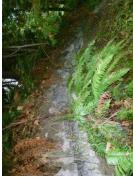
PHOTO 16 – Exposed dry laminated Silty Clay on ridge
