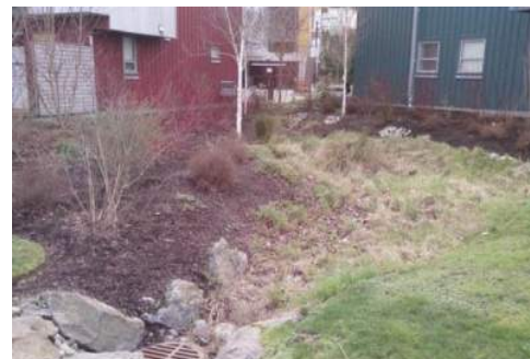
Rain garden adjacent to buildings.
