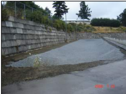
Surface Infiltration Swale
