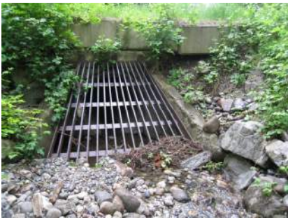
Shaw R4 (culvert inlet)
