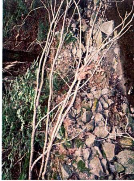
PHOTO 18 – Slide Scarp Below Residential Lot – Note Heavy Brush/Waste Covering Slope
