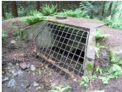
Briarwood R2 (culvert inlet)
