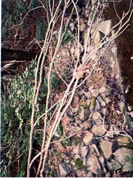
PHOTO 22 – Rip Rap Bank From Abandoned Road Crossing
