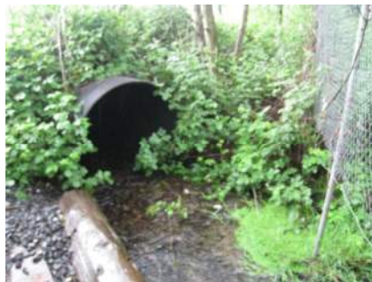
Watershed R1 (culvert inlet)
