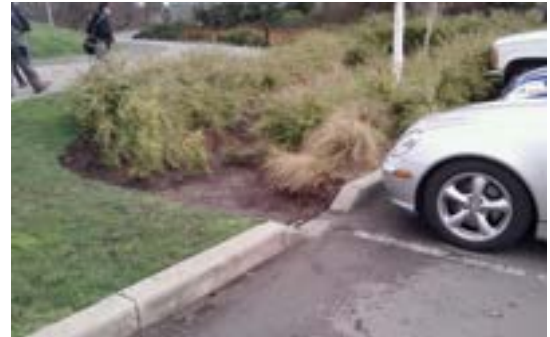
Rain garden adjacent to parking lot.
