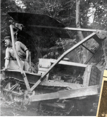
George Watkins and his bulldozer clearing brush 1952.
