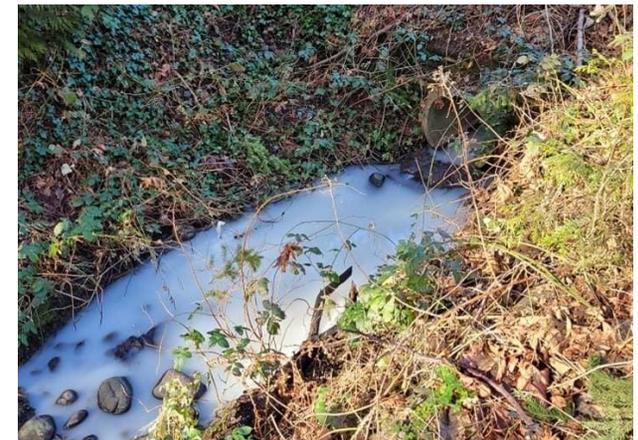
**Improper disposal of paint washout in to a storm sewer connection results in contamination a local creek.**
