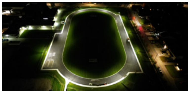
Delta Secondary School Track and Field Renewal
