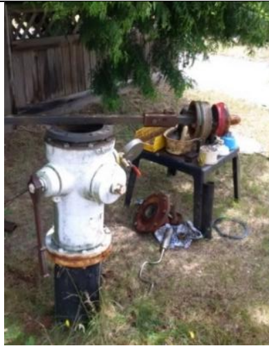
Figure 15: Fire Hydrant Undergoing Regular Annual Maintenance
