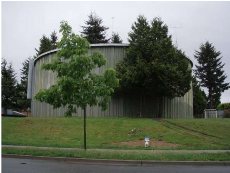
Figure 13: Hellings Reservoir in North Delta
