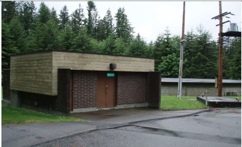
Figure 10: Water Reservoir and Pump Station on 64 Avenue
